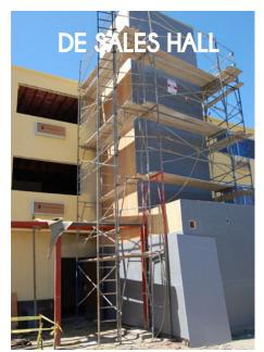
1/4 inch fire-shield sheathing screwed to the 3/4 inch plywood
