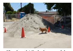
Pile of sand: NB: the bottom of the electrical conduit trenches, there must be 6 inches of sand mixed with pee grave as a base for the conduit pipes another 6 inches on top of the pipes before the back fill takes place
